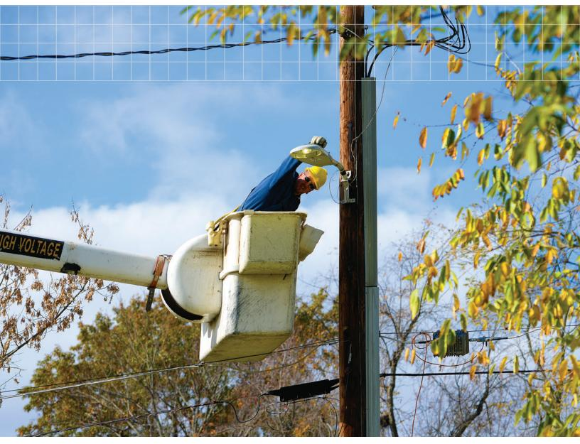
Several participating AMP member communities have upgraded to higher-efficiency street lighting through the Efficiency Smart program, which provides rebates on top of the cost savings from reduced power use. Shown here is a Georgetown Electric Department crew working on an LED street lighting project completed in 2014.
